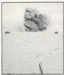
1st Bn. combat engineers shooting line charge into first minefield inside Kuwait. The charge is a chain of 1,100 pounds of C4, rocket-assisted. Photo: 1st Lt. Brian Hormberg
